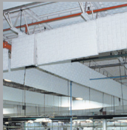
Wall-to-wall cable mount
