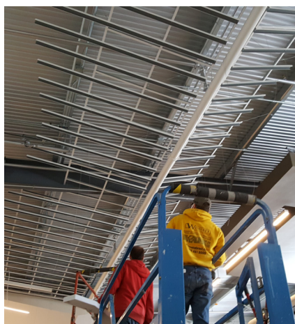
Raft Installation Example
