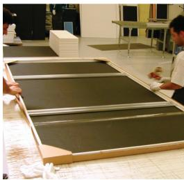
Atop the back of each BALANCE Ceiling Cloud's width there are two aluminum strong-back channels.
